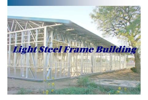
Light steel frame building in Botswana is one of the most exciting developments in the building industry. This method of building has been used in the US, Europe and Australia for decades but has only recently been introduced here. It offers quality, cost efficiency and speed of erection for low-rise and double storey residential and non-residential buildings. Many of the hotels currently under construction in South Africa to cater for the 2010 world cup are being built with this system.
